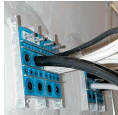
**EN** The Roxtec B frame is a flanged, bolted together metal frame. Frame parts are assembled to make different sizes and combinations of openings. Suitable for installation also around existing cables and pipes.
